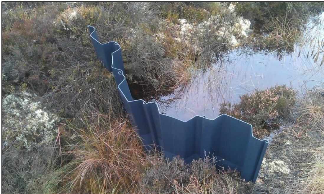
Plate 2-3. Example of plastic dams to be used for on-site drain blocking where peat dams are not suitable.
